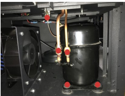
Remove pipes and screws
