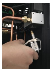
Cleaning before installation
